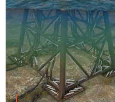
130 km of 220-kV subsea cables connect the MOG to the Stevin high-voltage substation in Zeebrugge.
